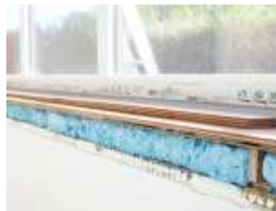
Insulation of window & door frames outside
